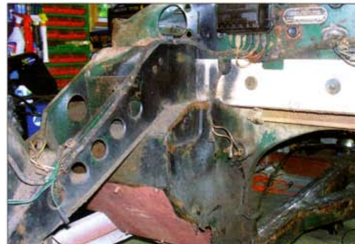
Removing all of the bolted-on body panels, interior and drivetrain gave Peter a good look at the car's condition. After beginning repairs, he decided not to try to reuse the original frame.
